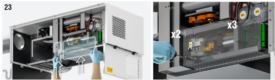
Fig. 23. Refit the plexiglass panels.
